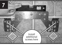
Level the bracket then mark, drill and install two additional plastic anchors and screws. If pre-existing bearing rods can be used, screws are not necessary.
