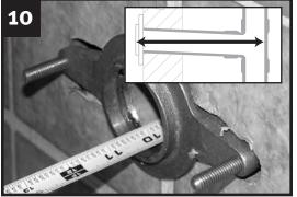
Determine the drain nipple depth by measuring the distance between the back of the sanitary tee (or elbow) to the front edge of the brass flange.
