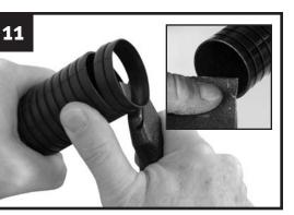
Cut the tube at the groove using a sharp utility knife to ensure a square, flat cut. Clean burrs from the cut end with emery paper.
