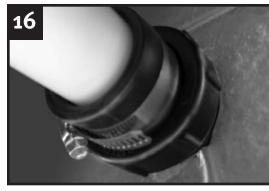
Tighten the compression nut and gear clamp.
