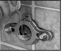
Clean face of existing wall flange then install the brass flange with the clear inspection disc. Slowly pour water into the drain.
