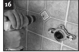
Drill holes for the lower anchor screws and insert plastic anchors.
